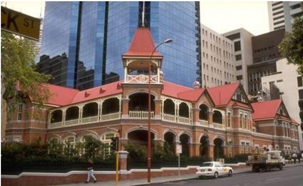
The Weld Club, Barrack Street Perth (Conservation Plan, John Taylor Architect, 2002).
