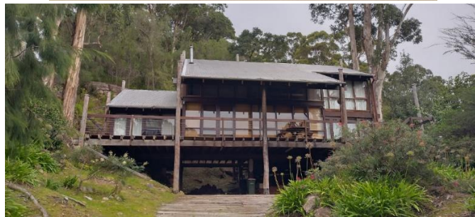
50 Riverside Drive Nornalup (sketch courtesy Jane Deykin, photo Brad and Ross Minchin).
